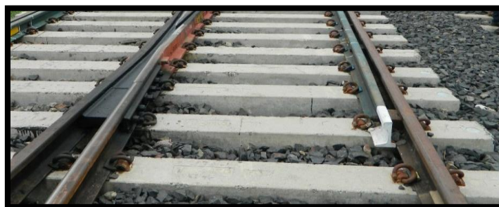
FIGURE NO. 3 GAUGE DISTANCE OF PERMANENT WAY
