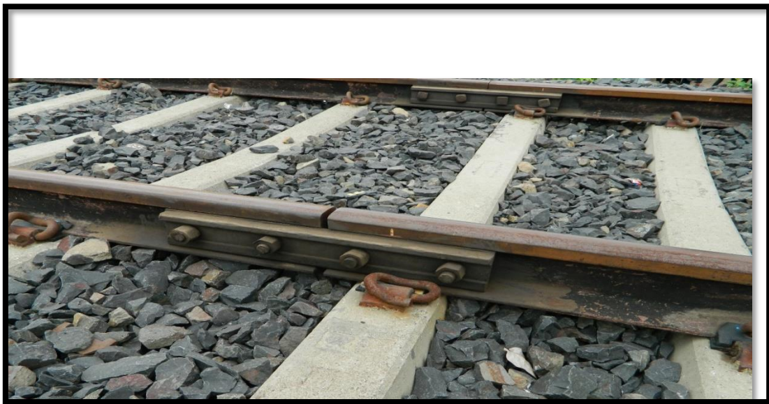
FIGURE NO.4 RAILWAY FIXTURES AND FASTENING
