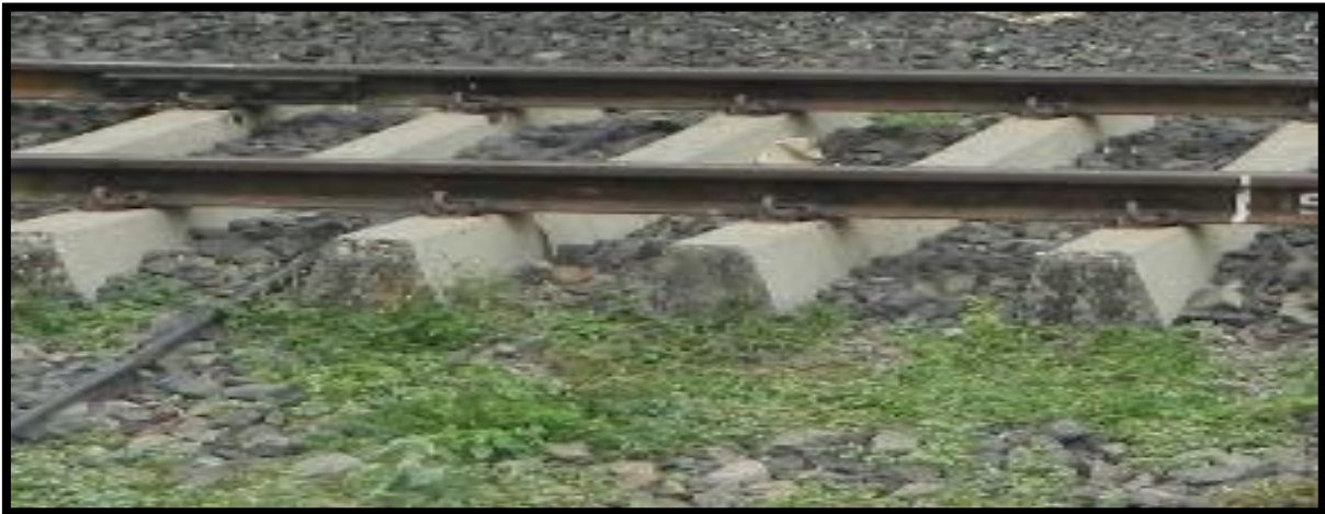
FIGURE NO. 5 RAILWAY BALLAST AND SLEEPERS
